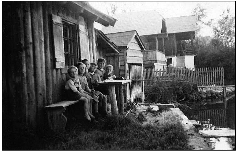
Boathouse, pier and laundry place in back of barn.
