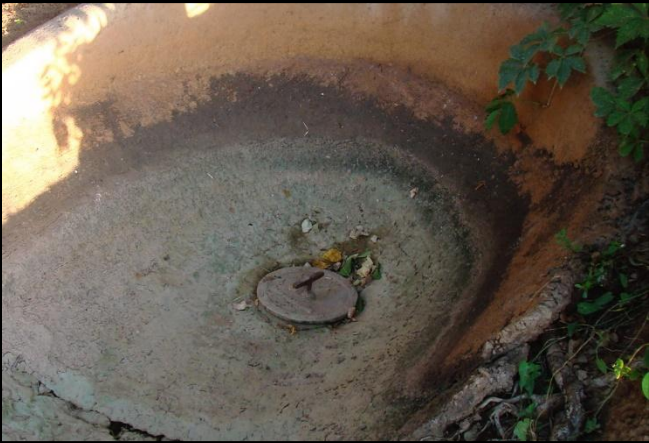
Gates are set to direct the water to desired home.
