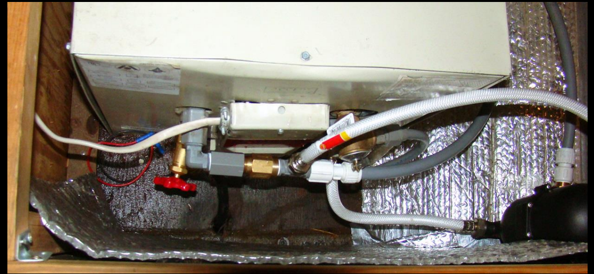
Installed a water system winterizing kit, allows charging system with antifreeze
